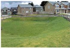
Also referred to as a dry extended detention basin, infiltration basin, wet pond, and retention basin
